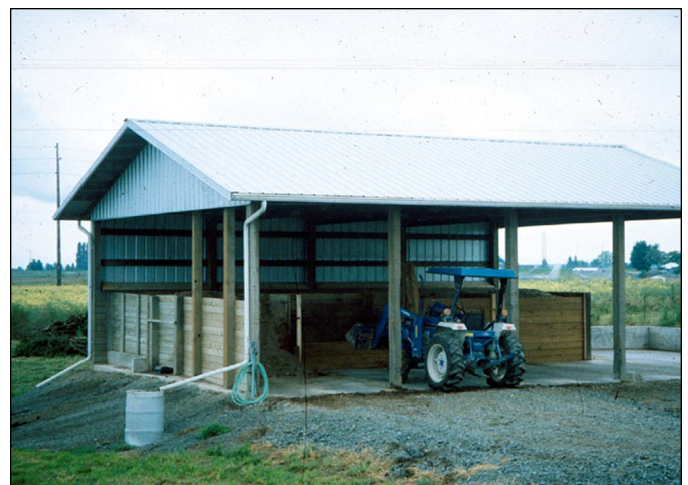
This roofed composting facility can be managed with a small tractor and front end loader. Note the roof runoff system that directs water to areas protected by gravel or grass and catches water for other uses.
